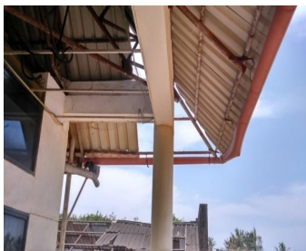
Part of roof blown away as of 2-6-2016
