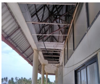
False ceiling blown away as of 2-6-2016
