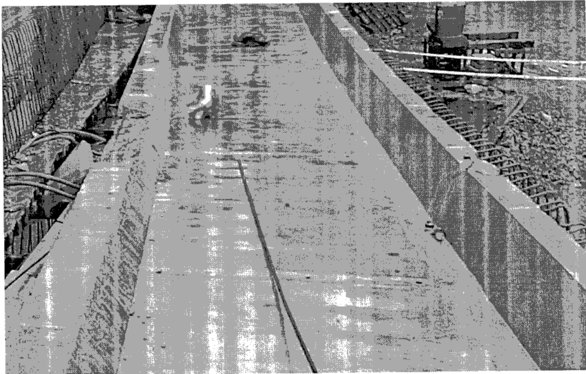
Photo 4 : Cracking and bending of the girders due to fall
