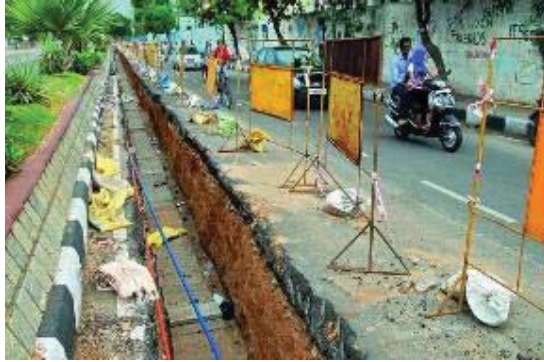
Figure 9.1 road cutting for utility laying
