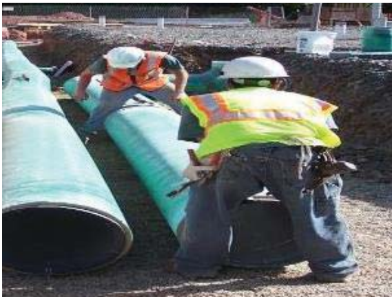
Figure 9.3 Utility cross duct
