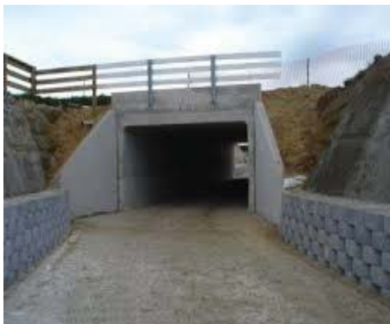
Figure 8.5 Culvert with abutment
