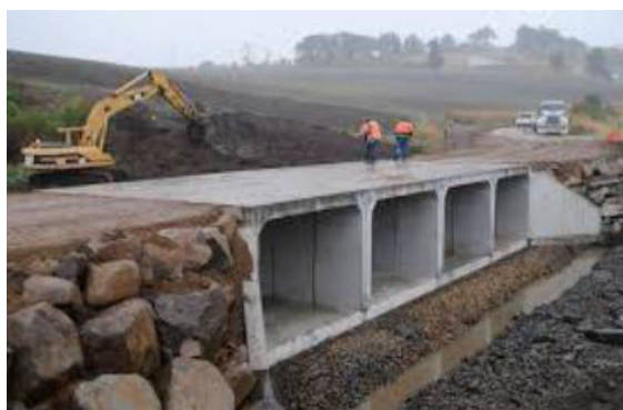
Figure 3.18 Multi-celled box culverts
